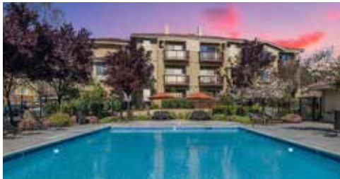
Multifamily Housing in San Ramon
