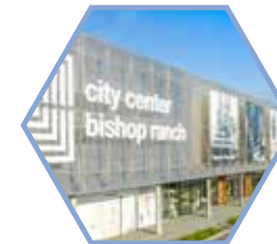
Completion of City Center at Bishop Ranch
